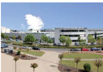
MEISINGER Headquarters Neuss, Germany
